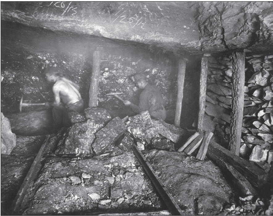
Figure 5 Photograph of mining at the face in an early longwall mine. Note the rock support on the right side of photograph. These mines operated from the 1870s to 1951 in fifteen counties. Most were located in the northern counties from Bureau through Will (fig. 2).
