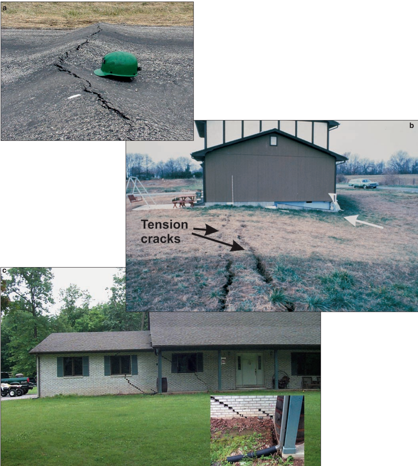
Figure 14 Photographs illustrating the sag subsidence event and features shown in figure 13. (a) Compression ridges formed in the road (feature R) as the result of ground movement (compression) associated with coal mine subsidence. (b) Tension cracks form in the ground surface extending through a home (feature H1); the foundation has settled at the house corner close to the center of the sag. (c) The brick-sided house (feature H2) in the tension zone shows downward bending (compare roof lines). The left side of the home is closest to the sag center and has dropped down. Insert: Ground has pulled away from the porch toward the sag center (left).
